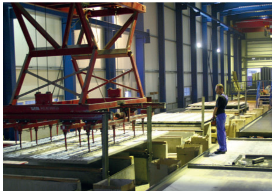
Fig. 2: Stacking stations for floor slabs
